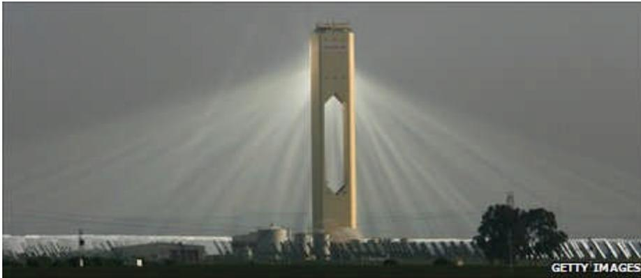
The PS10 solar tower plant near Seville, Spain. Mirrors concentrate the sun's power on to a central tower, driving a steam turbine
