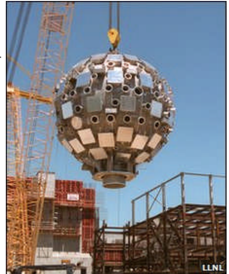
The 130-tonne target chamber is kept under vacuum for the experiments
